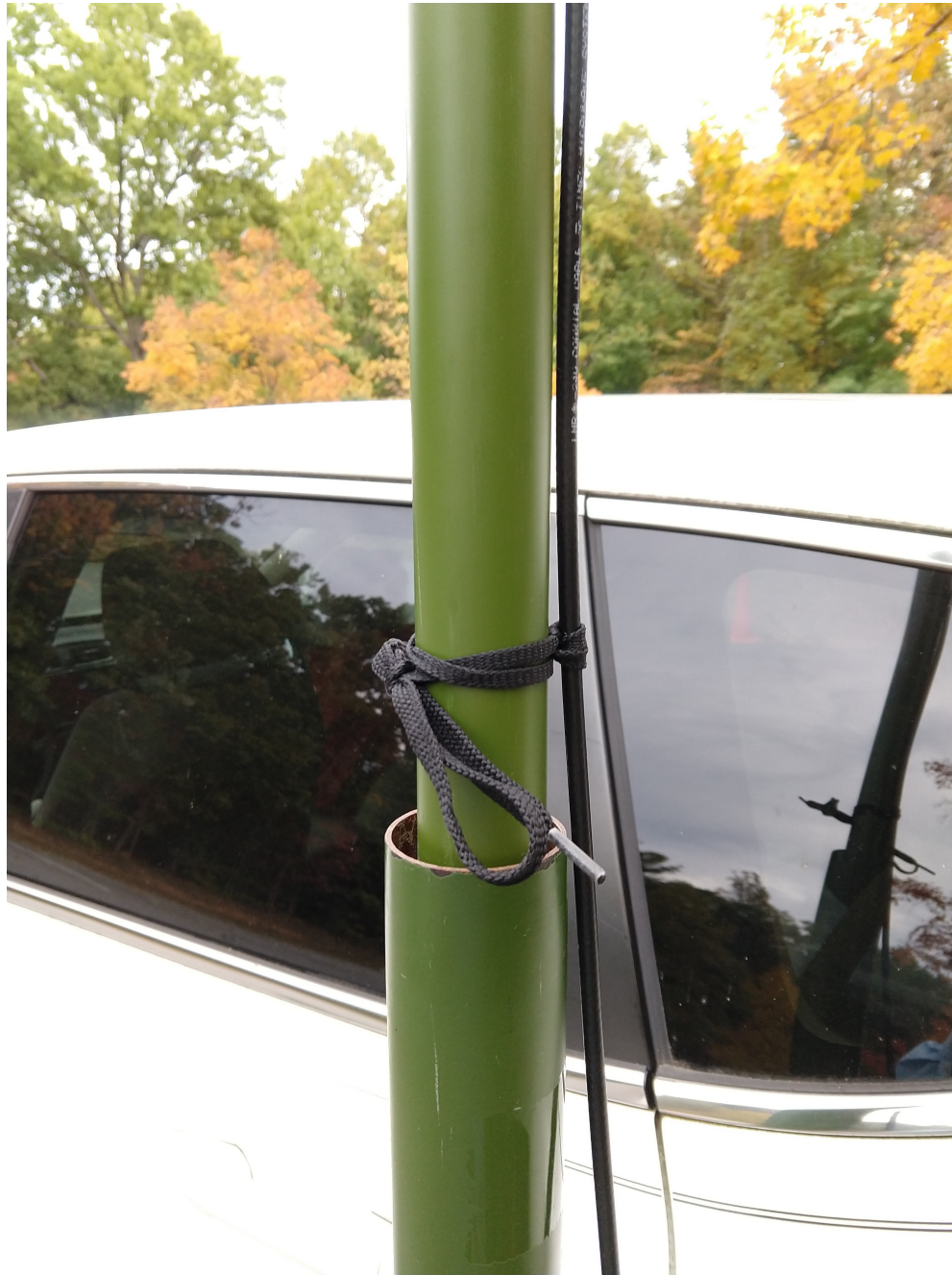
coax cable secured to each mast segment
